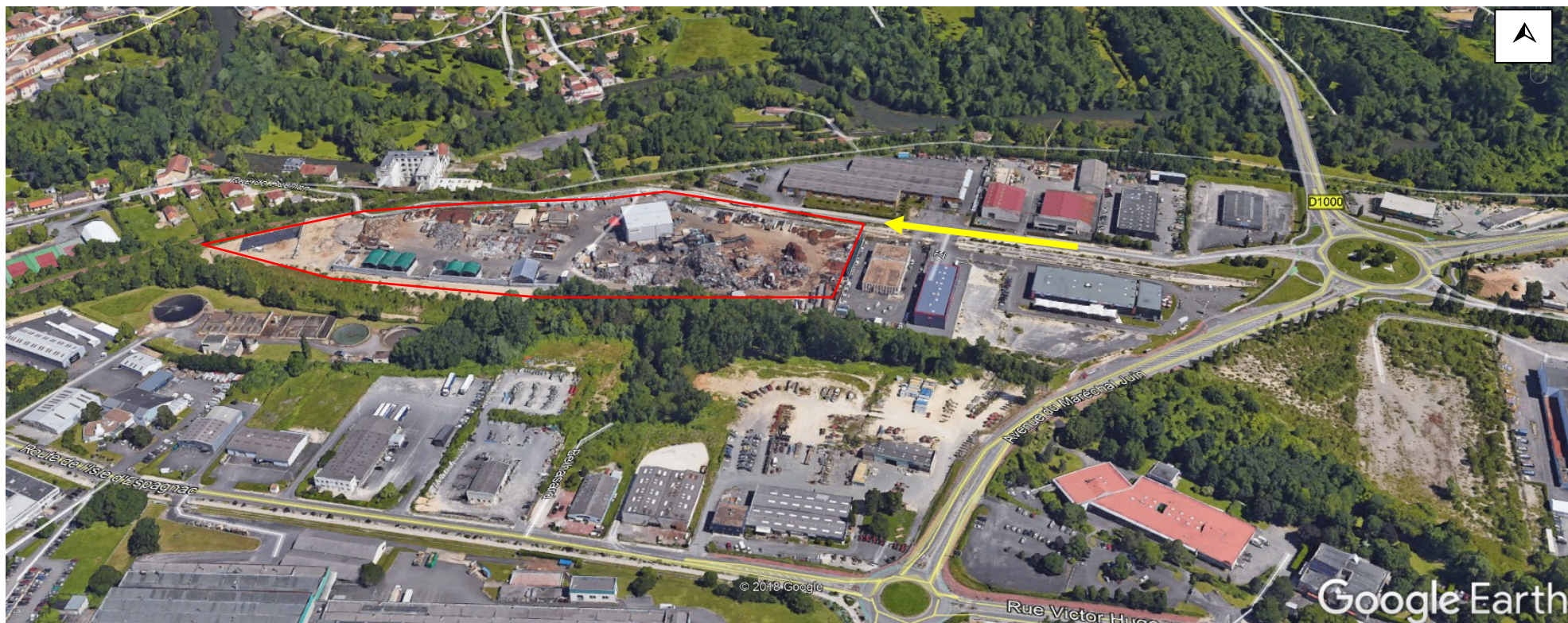
FIGURE 9 : VUE AERIENNE SITE SIRMET 16 (DATE IMAGE SATELLITE : 20/04/2017 – GOOGLEEARTH)
